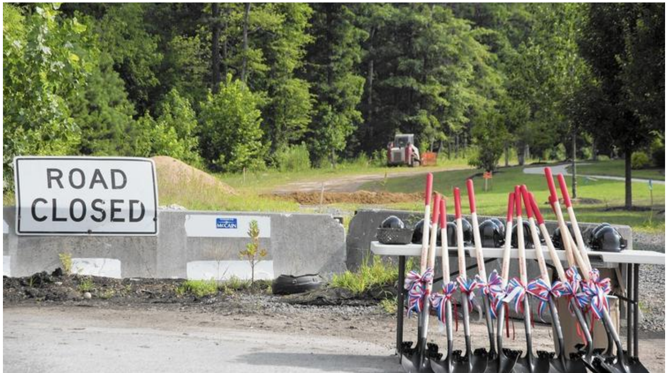
Shovels are lined up for the ceremonial groundbreaking on what will become Town Center Boulevard in Odenton. (By Joshua McKerrow / Capital Gazette)
